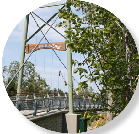
Elbow River Suspension Bridge
